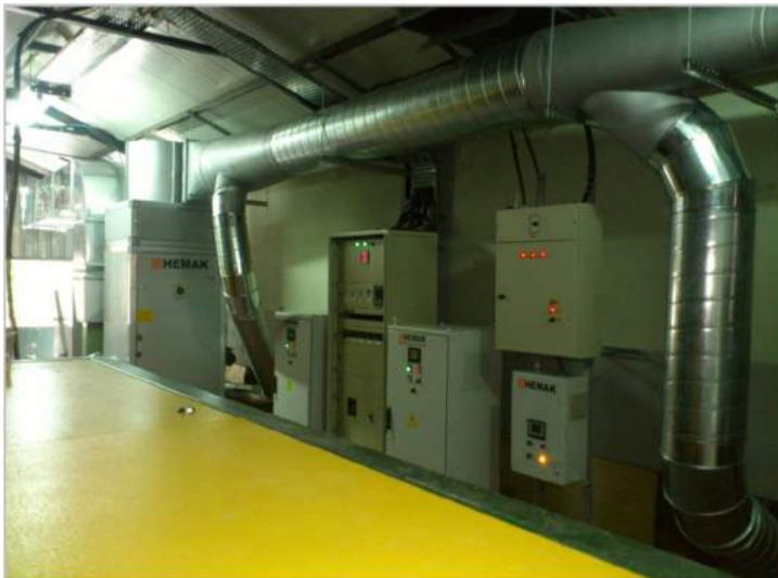
Equipped With Products Of World Famous Brands, Hemak Automation Panel Provides 100% Protection For Your Motors, Does Not Cause Any Malfunction And Does Not Require Maintenance.
