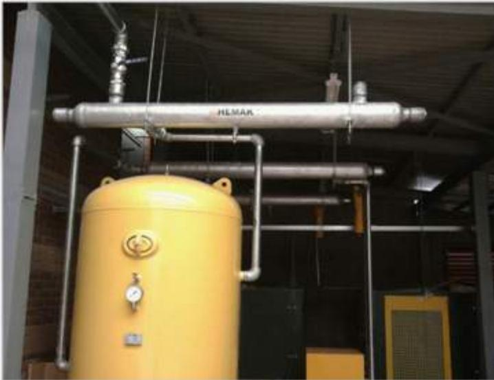
Galvanized Collectors And Compressed Air Preparation.
