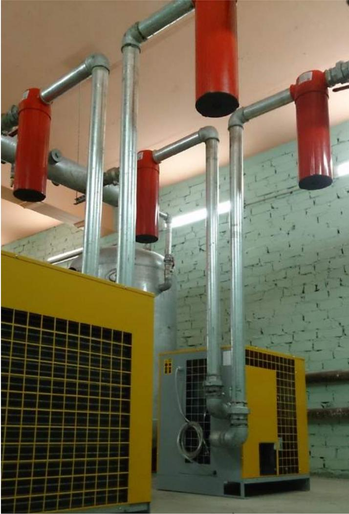
Seperator Collectors, Filters, Dryers and Tanks.
