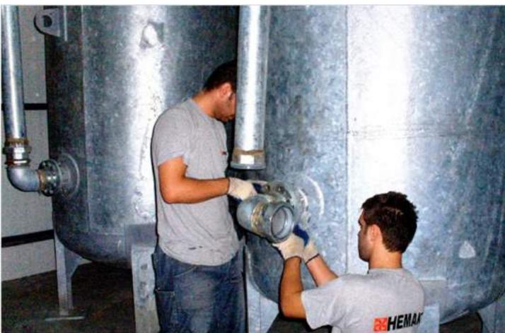
Galvanized Air Tank 4 " Connections.
